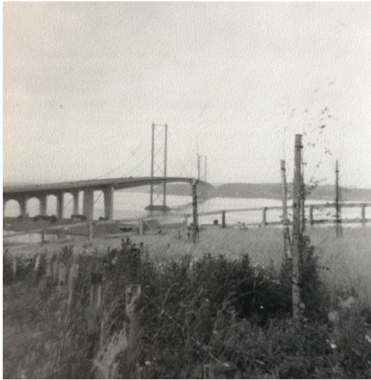
Forth Road Bridge
