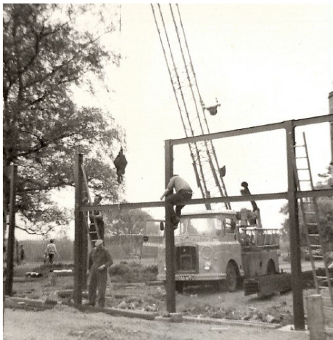
The new dining room under construction
