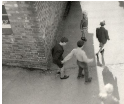
View from upper classroom
