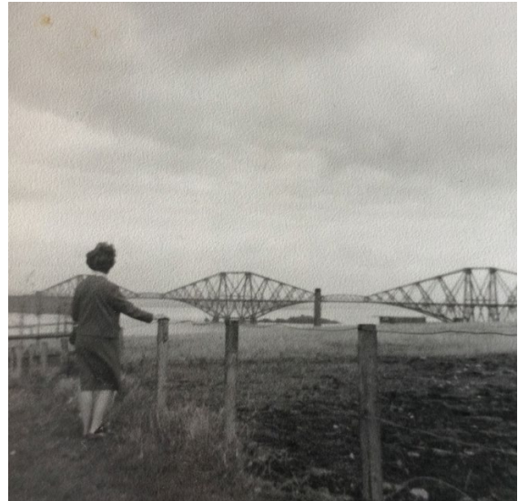
Forth Railway Bridge
