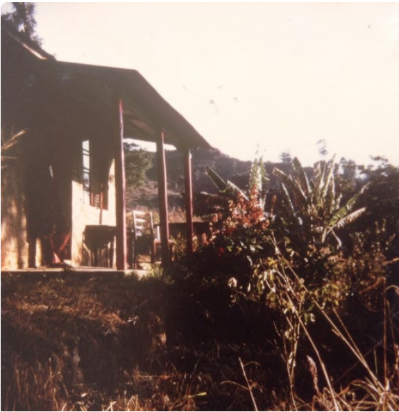
Left: View along the front verandah
