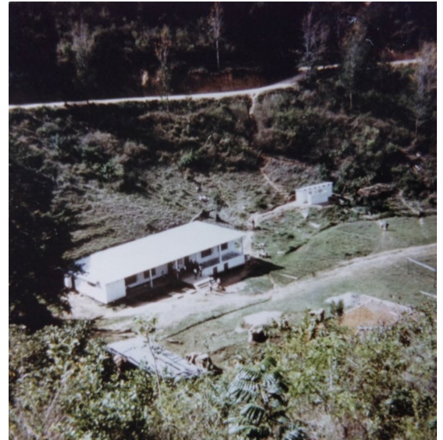
Right: Mgalu High School, set in the floor of the valley. Main building, with staff room and library (far left), Form I (middle) and Form III (right). The foundations for the new school building can be seen in the foreground
