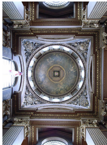
Ceiling under dome
