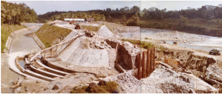
Construction of Headworks: Mataram Canal offtake from Kali Progo River (note temporary diversion)
