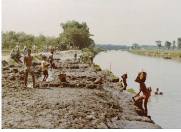
Removal of silt from river bed using porous silt buckets. Sandy silt is gathered from river bed in buckets by labourers who dive underwater. Buckets are carried on shoulders up steep banks (using ladders) then emptied. Other labourers ferry dry silt to nearest point accessible to lorries.
