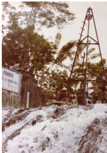
Borehole drilling (weir is scoured)
