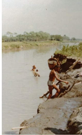
Removal of silt from river bed using porous silt buckets. Sandy silt is gathered from river bed in buckets by labourers who dive underwater. Buckets are carried on shoulders up steep banks (using ladders) then emptied. Other labourers ferry dry silt to nearest point accessible to lorries.
