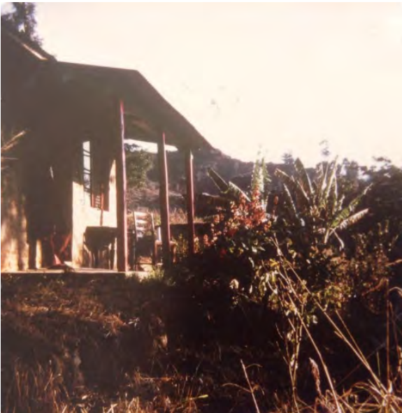
Left: View along the front verandah
