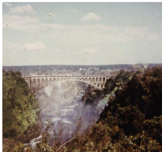
Right: Rhodes Railway Bridge, linking Zambia (left) to Rhodesia (right) – notice the train on top
